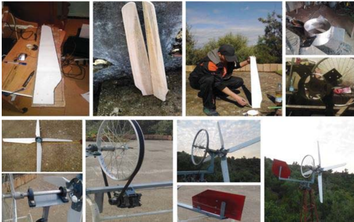
Fig. 6 Realization steps of the designed wind turbine.
